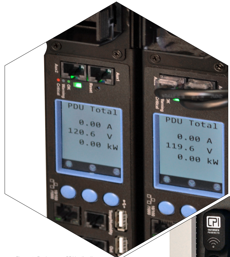
Figure 8: Rack-mount PDUs distribute power to equipment within the enclosure and can provide remote power monitoring and outlet control. Photo of CPI Switched Pro eConnect® PDUs.
