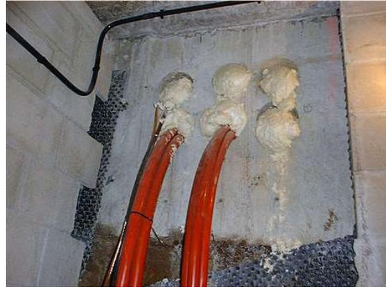
Figure 7. Silicone and foam used to stop water ingress
