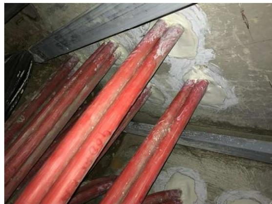
In this scenario, ducts, vaults and maintenance holes fill with water and debris, where cables and equipment can be exposed to high levels of water and humidity. This is the highest risk scenario and is very common when construction specifications do not include details for sealing ducts and building entries.
