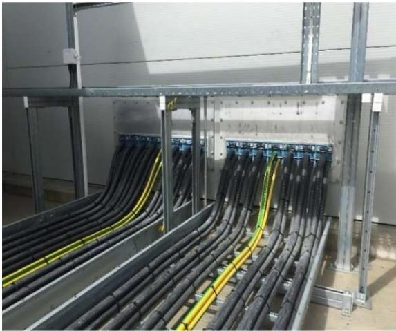
Figure 10. Large area building penetrations for power systems sealed against water ingress
