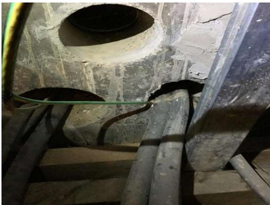
On-site remedies vary, but most commonly, foam or silicone is used (Figure 7). While these remedies will provide some level of protection, they are not effective long-term at stopping water pressure that builds up behind the seal.
