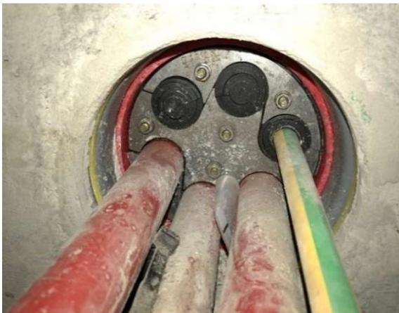
Figure 8. Mechanical seals for fiber and power vaults. Purpose built seals that provide long term protection against water ingress
